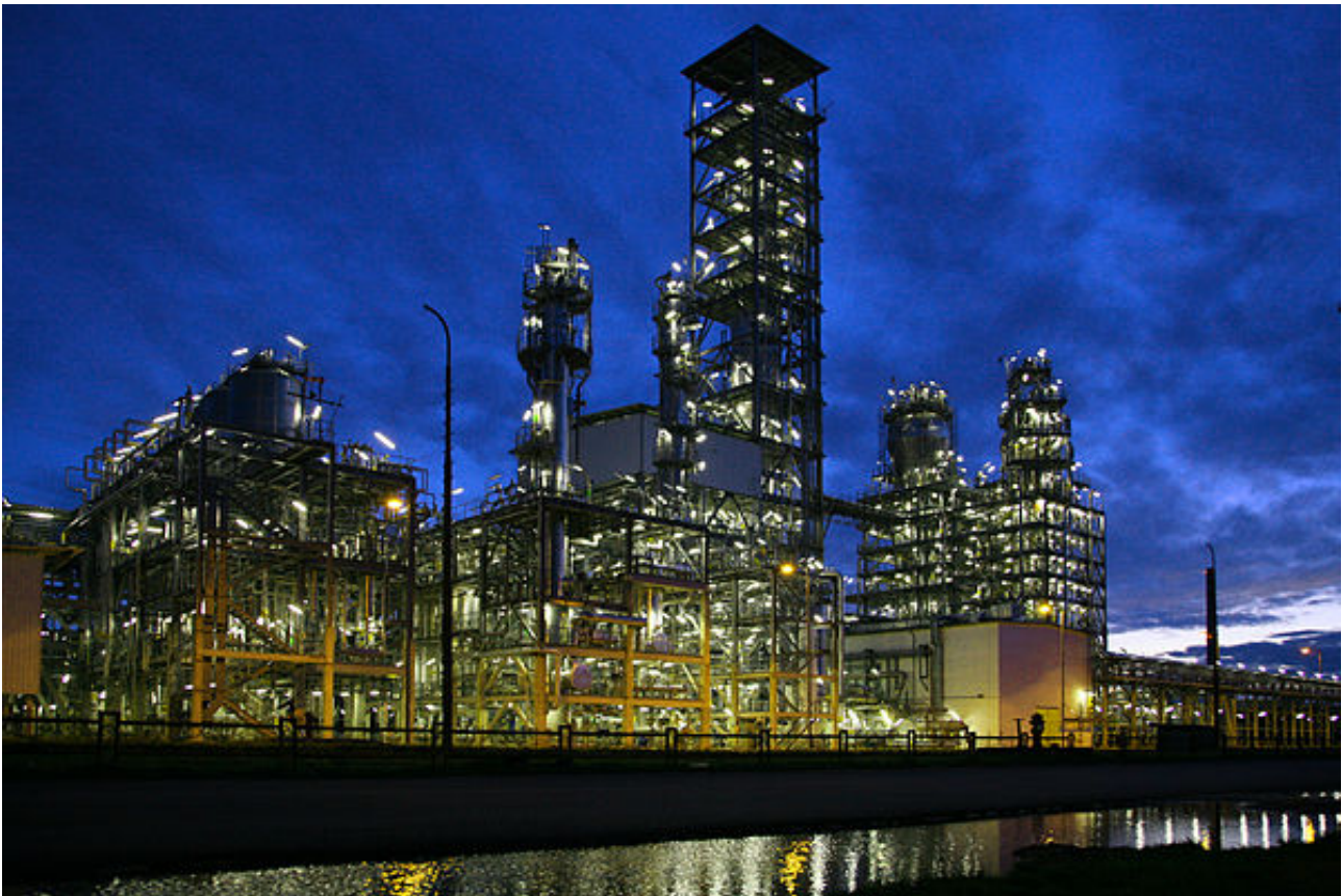
New polypropylene plant PP3 in the Slovnaft oil refinery ( Bratislava , Slovakia)
